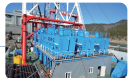
Mixer Plant Operation Room
