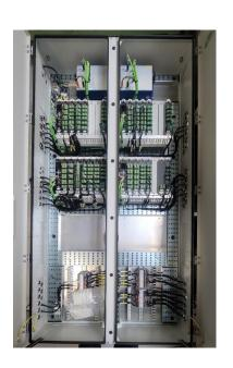
Engine Control System Cabinet / Cylinder Control System Cabinet / Second Fuel Engine Control Cabinet
