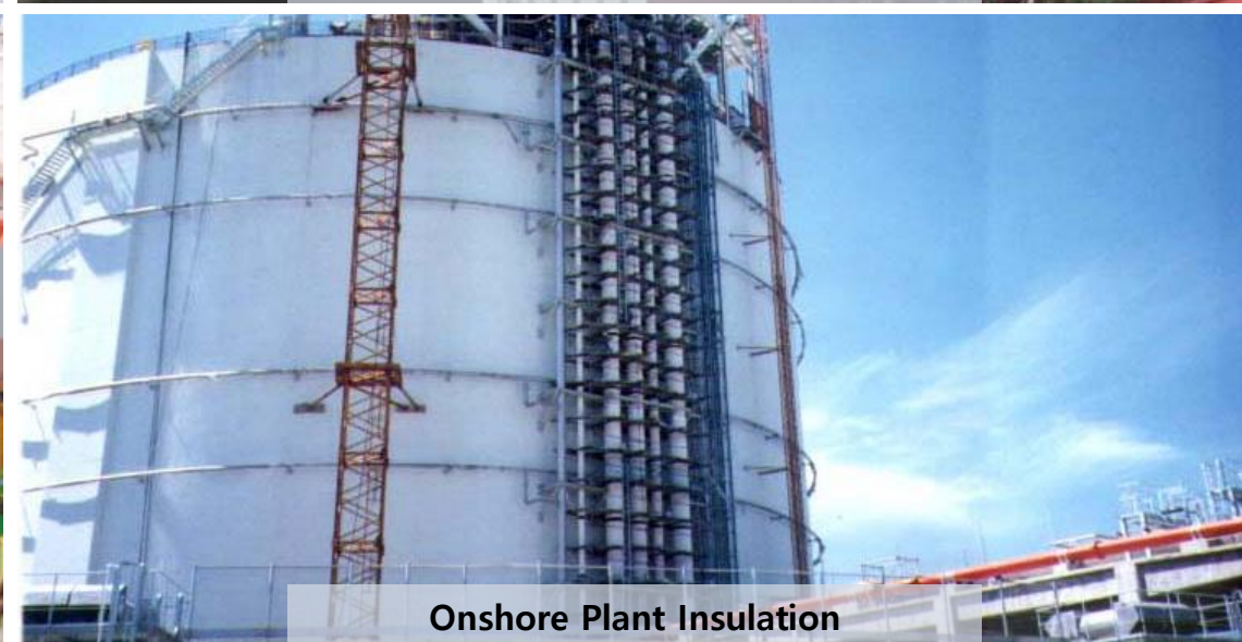
LPG Tank Insulation(Spray)
